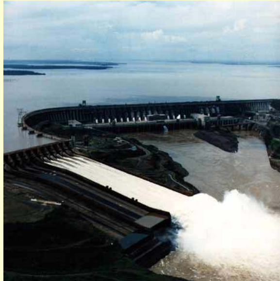
Hydraulic jump below the spillway (水壩洩洪道)
